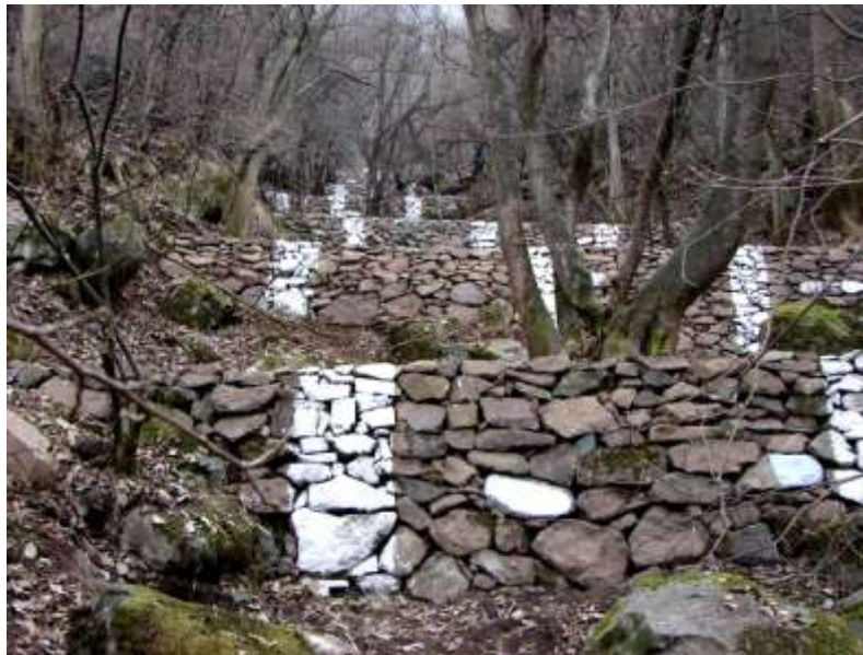
Check dams to control water flow
